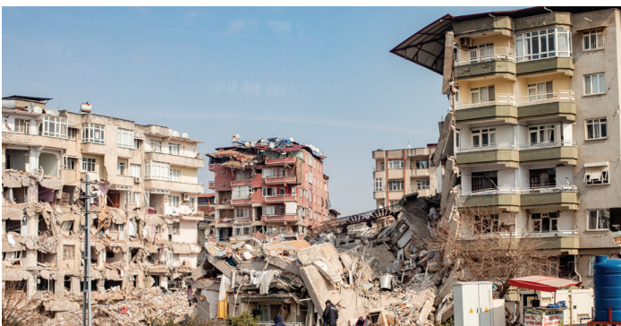
Destroyed buildings in Antakya, Hatay, February 2023
